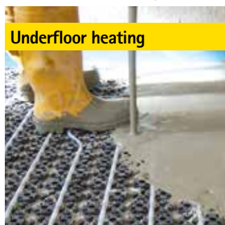
Floor smoothing and levelling
